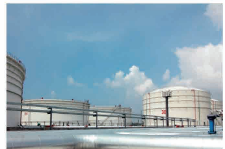
Industrial oil depot
